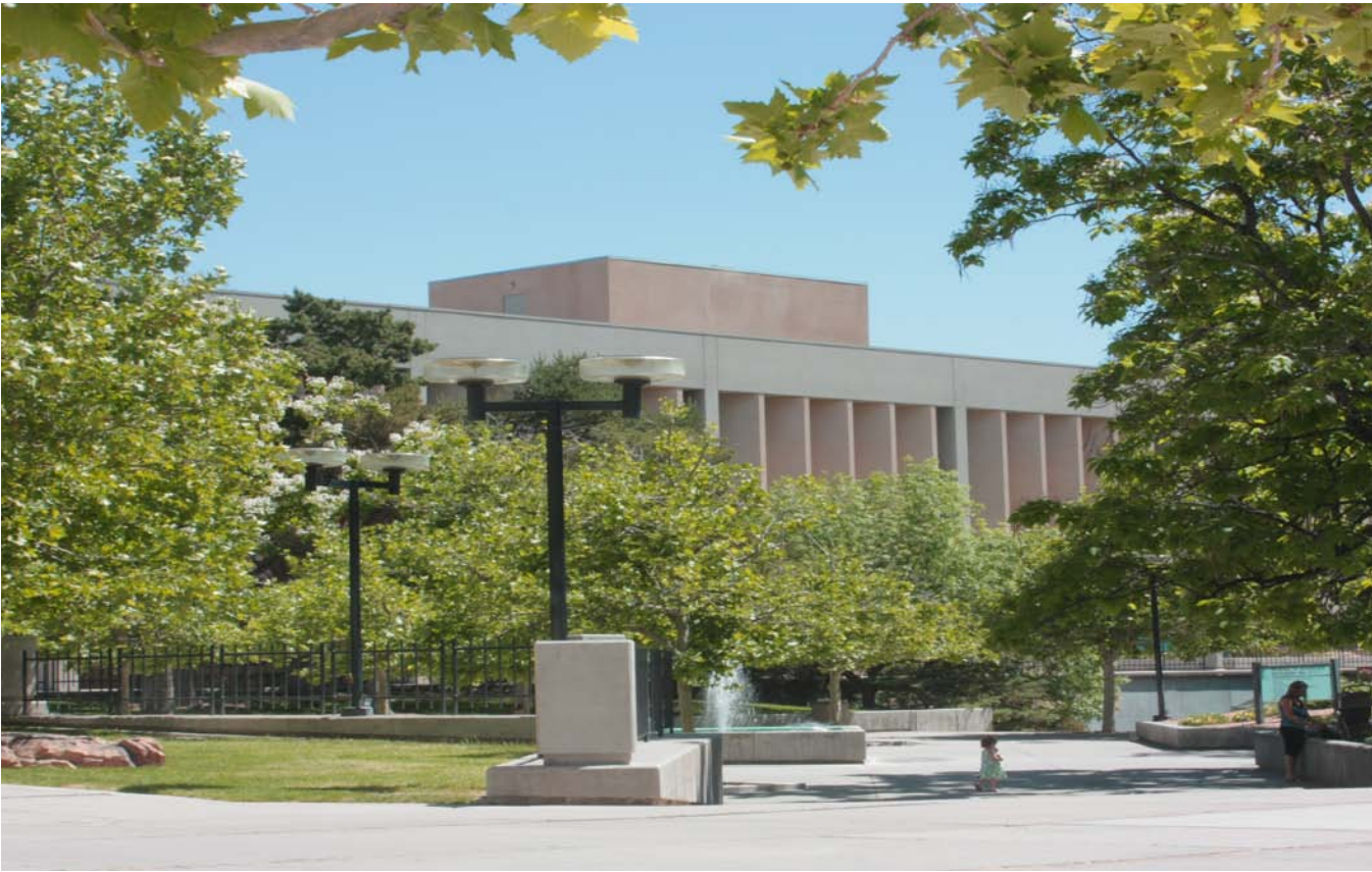
Former UNMHSC Cancer Research Treatment Center and Plaza
