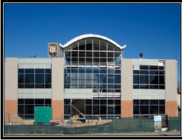
RIB Under Construction
