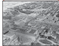
Aerial view of North Campus.
