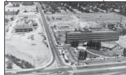
Aerial view of Basic Medical Sciences Building construction.
