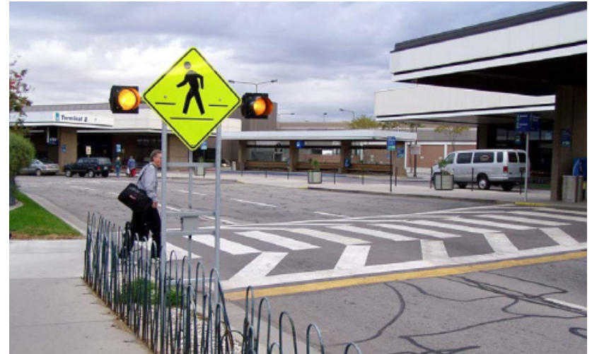
Figure 5 A Federal Highway Administration survey found that raised crosswalks increase pedestrian visibility and the likelihood that a driver yields to pedestrians, especially when combined with a flashing overhead light.
