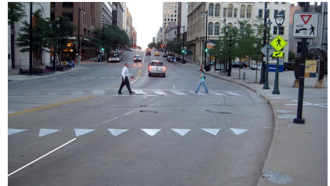
Figure 2 An advanced yield line (“shark teeth”) and yield sign alert drivers to the upcoming crosswalk and encourage them to slow down.
