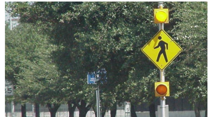
Figure 3 A pedestrian crossing sign with a flashing beacon. This sign makes it easier for approaching drivers to see an upcoming crosswalk. In some cases, the beacons are activated by the pedestrian pushing a button when they are ready to cross.
