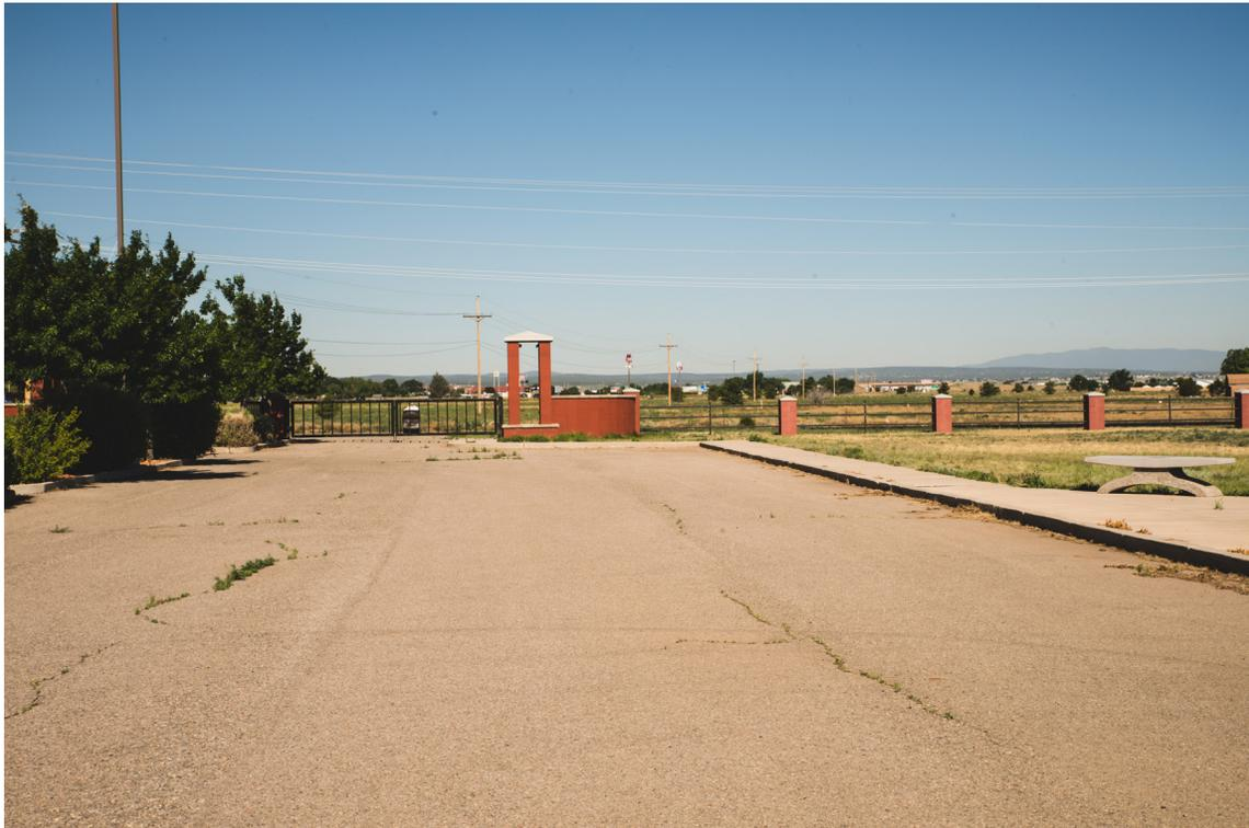
*Linear cracking evident on parking surface.*
